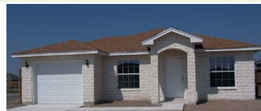
One of 14 Affordable Homes in Brownsville, Texas that Meet DOE's Builders Challenge
