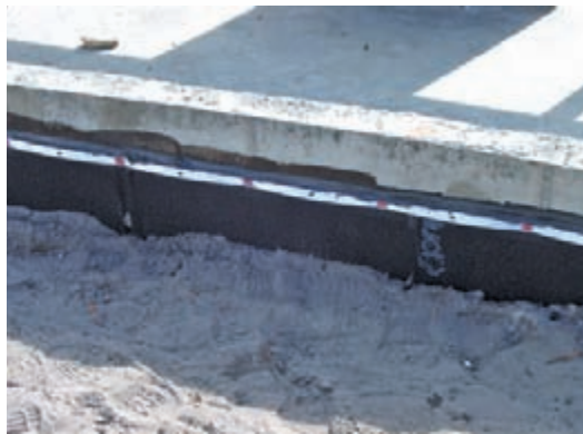
Extra measures were taken to ensure the foundation and shallow basement were waterproof.
