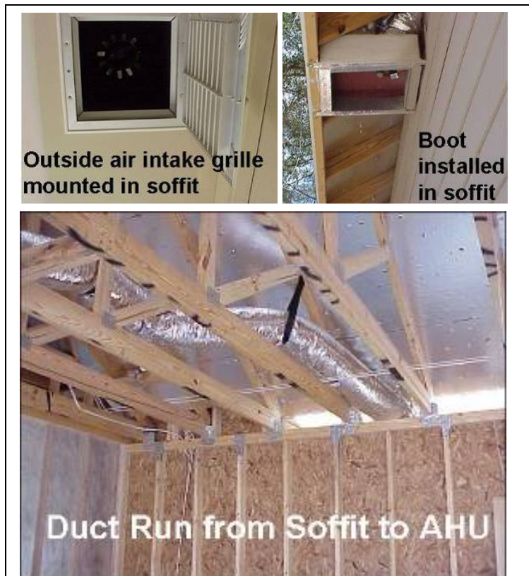
Figure 11 Outside air ventilation system details
