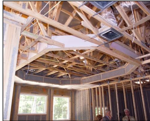
Figure 20 Solid blocking at tray ceiling framing as required by TBIC.
