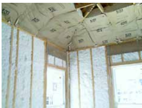
Continuous formaldehyde free fiberglass blown insulation
