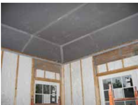
Sealed drywall at ceiling
