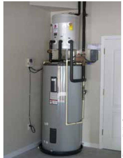
120 gallon storage hot water tank with drain back tank above
