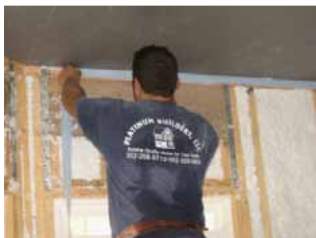
Foam gasket at ceiling/wall joints ensures airtightness
